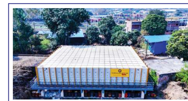
7,56,000 Litres SMC Panel Tank - Railway Station, Ludhiana
